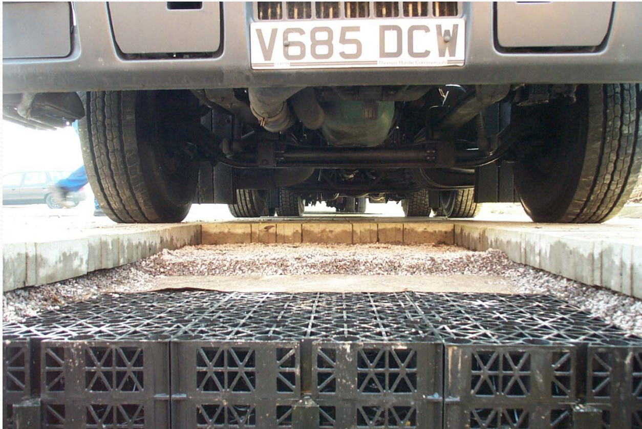
Is this strong enough? 40 tonne low loader parked on Formpave surfacing with 50mm bedding which is laid on the inner skeleton of Skeletank®
