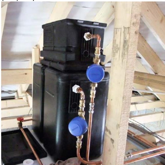
This is the Skeletank® pump sump unit with an integral overflow. The pump sits within the chamber. The pump we recommended has an internal pressure control which removes the requirement for a control panel in your house. The pump only works on demand.
