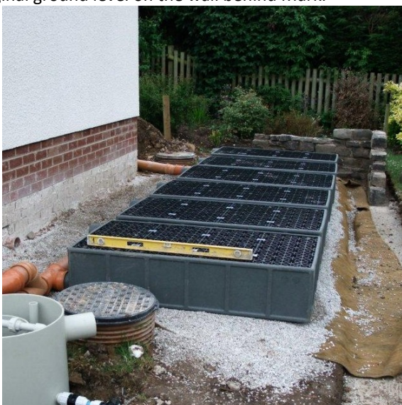
The rainwater storage units are laid level.
