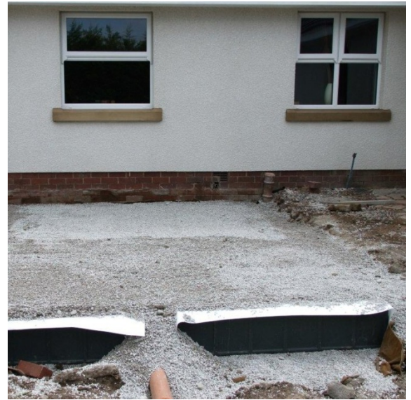
The top stone layer ready for the paving.
